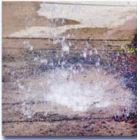
Misdirected sprinkler heads?
