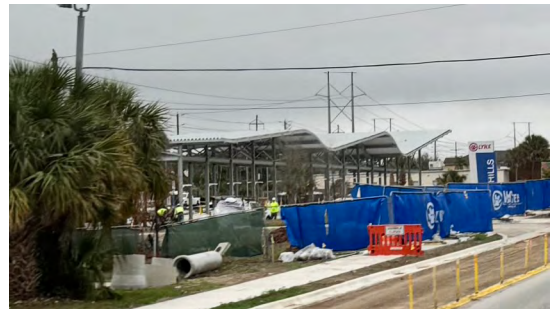
The LYNX Transit Center is nearing completion in Pine Hills.
