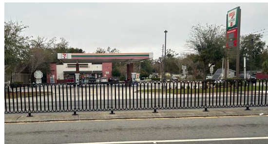
Median fencing was installed to prevent pedestrian crossings outside of crosswalks in Pine Hills.
